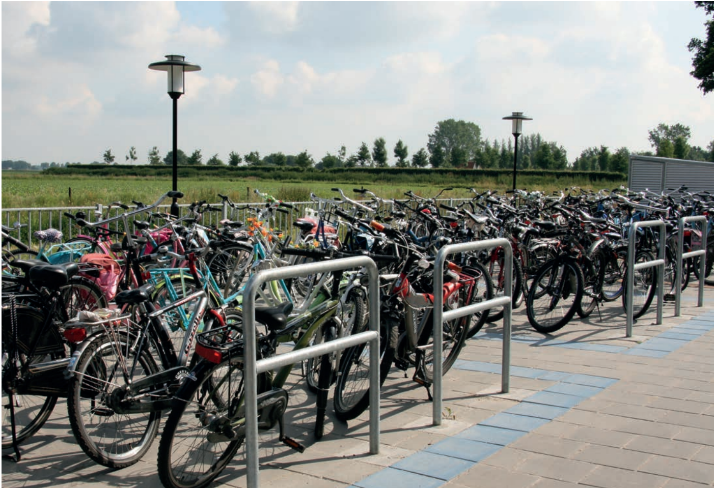
SHEFFIELD STANDS WITH CROSS STRUT (Ø41.5mm)
